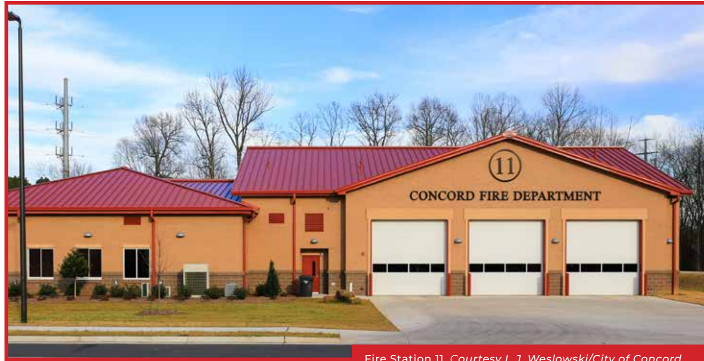
Fire Station 11. Courtesy L.J. Weslowski/City of Concord.
