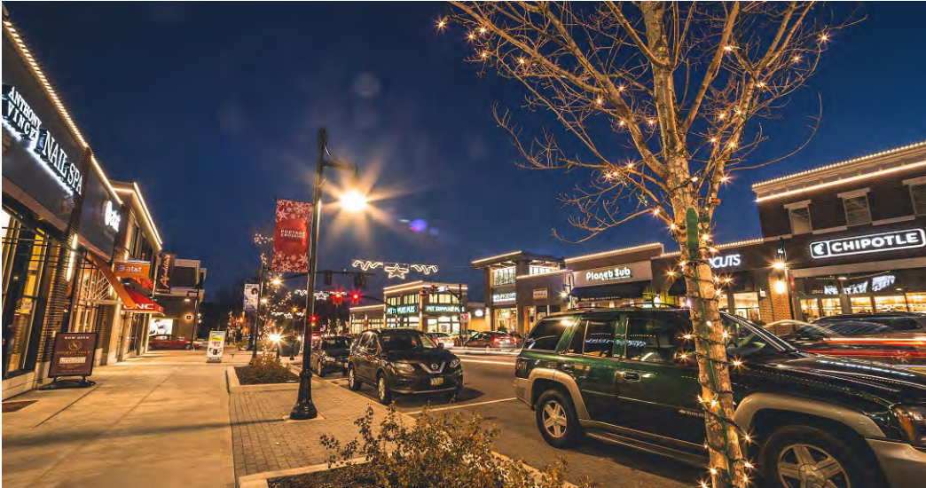
New development at Portage Crossing. Photo: City of Cuyahoga Falls.
